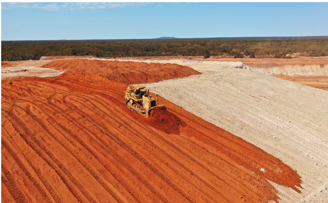
Figure 1: Dozer spreading topsoil on the Lost Dog waste dump on 25 Aug
