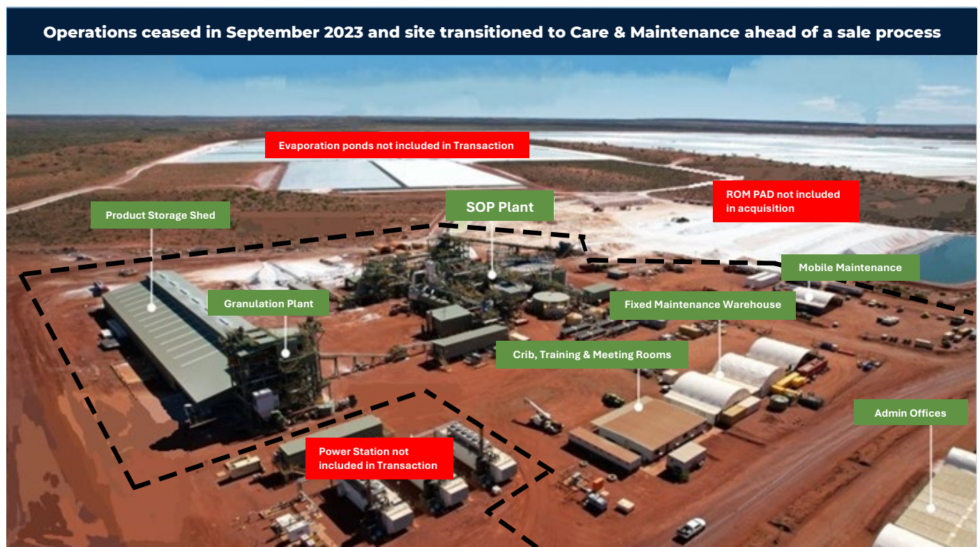
Figure 1 – Photograph of the Beyondie Potash Project in 2023 when in operation by Kalium. The Transaction comprises a fully constructed processing plant, site offices and maintenance infrastructure. Specific plant components include, KTMS crushing circuit, Kainite conversion circuit, column flotation circuit, liquor cooling heat exchangers, evaporative cooling circuit, product separation centrifuges, SOP recovery and granulation unit, RO water plant and a bulk storage shed.
