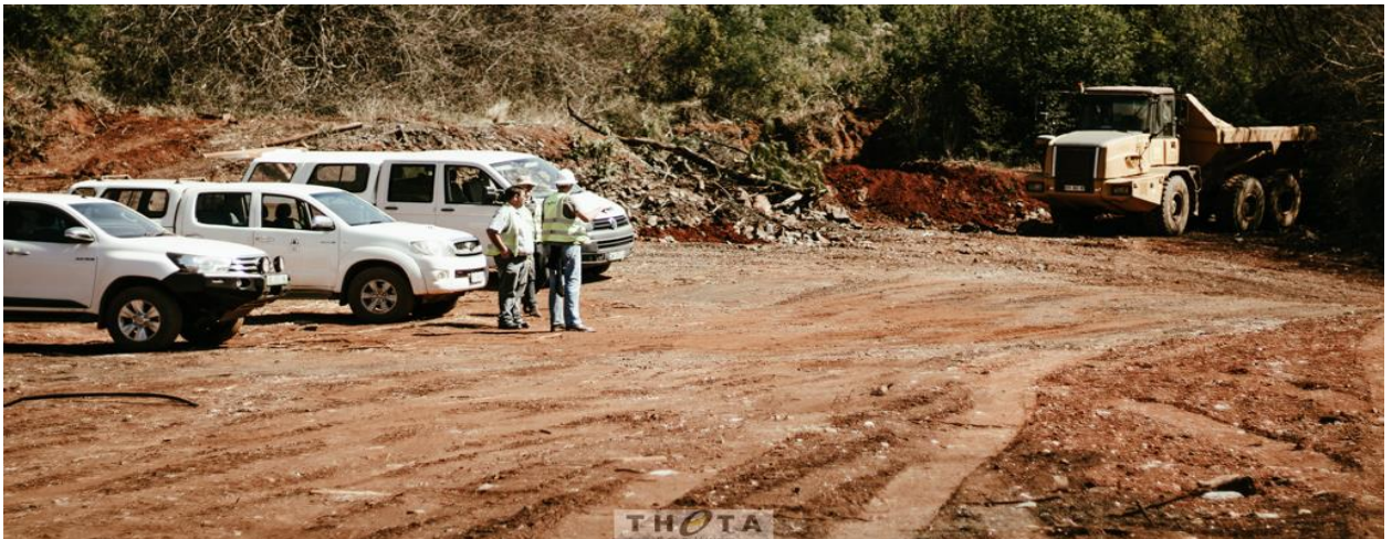
Figure 1: Plant site earthworks preparation for dolomite drilling
