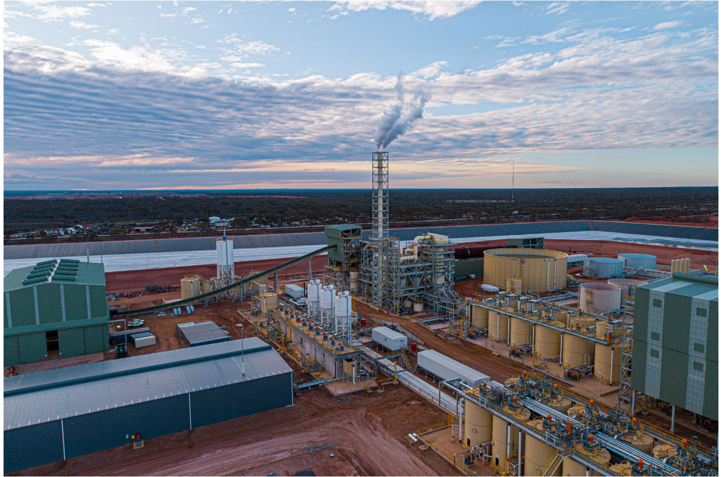
Waste gas treatment plant removes impurities from gas in the rotary kiln before being released as steam
