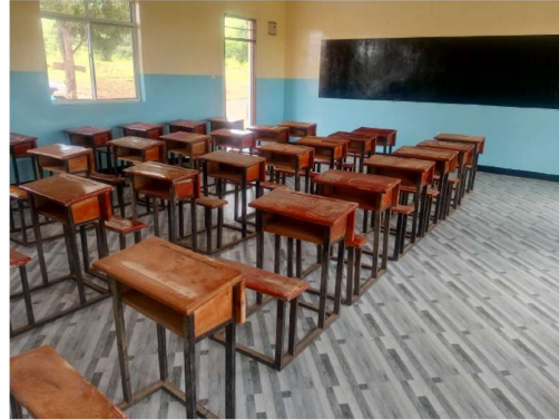
Completed high school classroom
