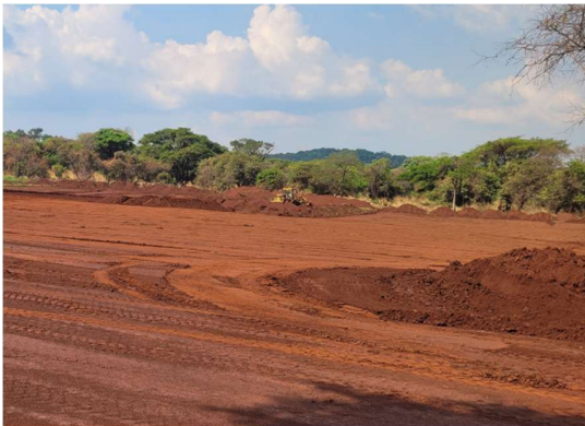
Establishment of equipment laydown area
