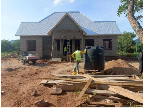
Police station under construction
