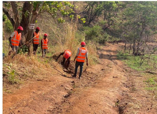
Development of access to planned mine pit area
