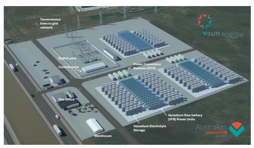
Example 50MW 10-hour (500MWh) VFB BESS Layout
